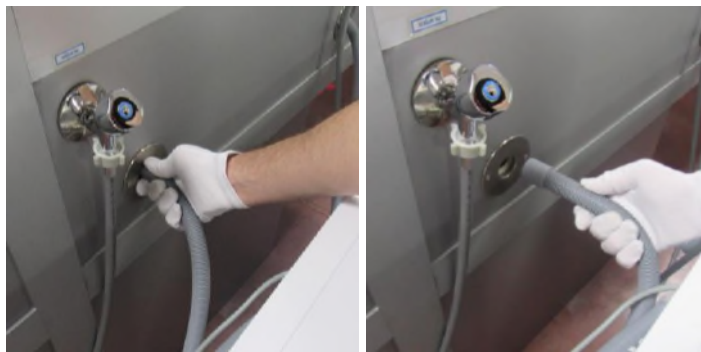
1.3 Disconnect the drain hose
